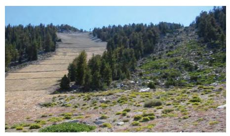
Side-by-side runs at Mt. Rose Ski Tahoe illustrate the two methods of cutting a run—the one on the left was graded by bulldozer and the other cleared by chainsaw.
