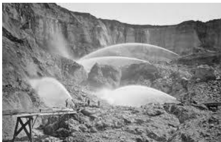
Figure 3. Hydraulic Mining for Gold and Minerals in the Late-1800s
